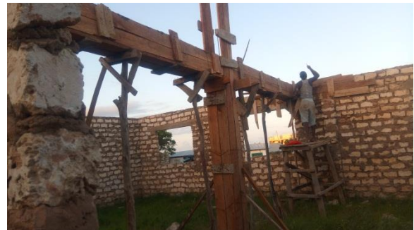
The beam is supported by the designed timber mold to shape the concrete mixture.
