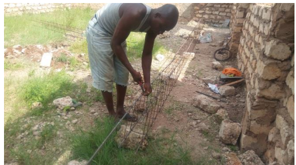
Binding the grills to strengthen the petition
