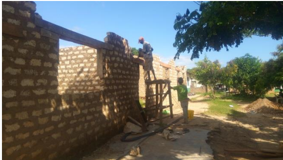
Pouring concrete in the fixed molder to support windows and door
