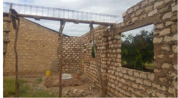
Mounting of the beam to support the concrete
