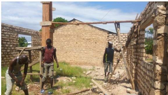
Building the central partition. Will also help in strengthening the structure.
