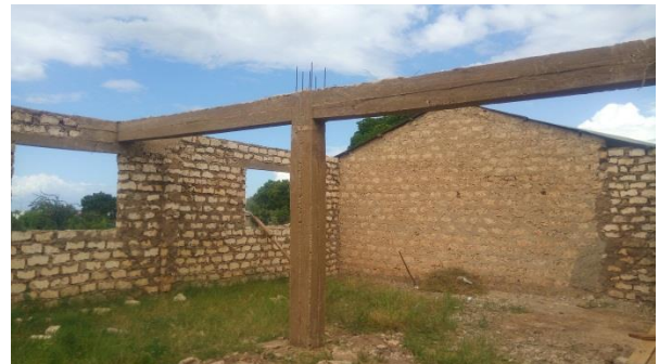
The final look after removal of the timber mold
