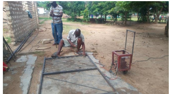
Cutting and assembling of materials ready to be welded.
